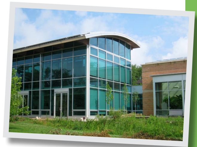
The Adam Joseph Lewis Center for Environmental Studies at Oberlin College in Ohio is one of many green buildings on college campuses.
